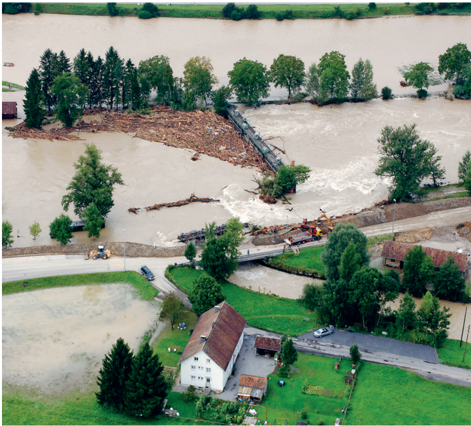
The flooded River Reuss in August 2005. A considerable quantity of large wood accumulated against the weir in Perlen (Canton Lucerne).
