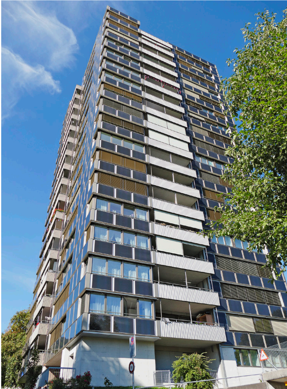
The photovoltaic facade of this skyscraper in Zurich Leimbach supplies around 85,000 kWh of power per year, covering a third of residents' energy consumption.
