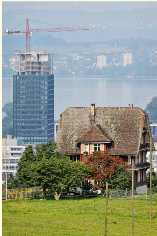
Building works on the tallest building in Canton Zug, Park Tower.
