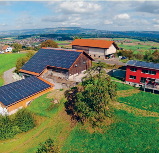
Photovoltaic system on the roof of a farm in Kallern (canton of Aargau).
