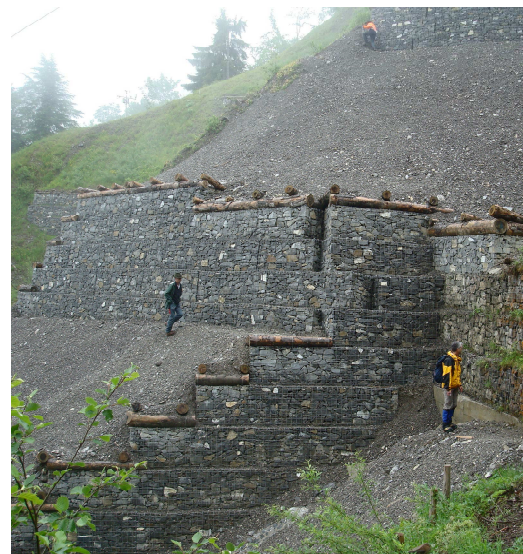
Ridge stabilised with gabion walls in 2011
