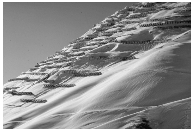
Figure 6. Supporting Structures in a Starting Zone on the Schiahorn Above the Town of Davos, Switzerland. A slab did release at the edge of the protected area, but could not develop into a large avalanche due to the supporting structures.
